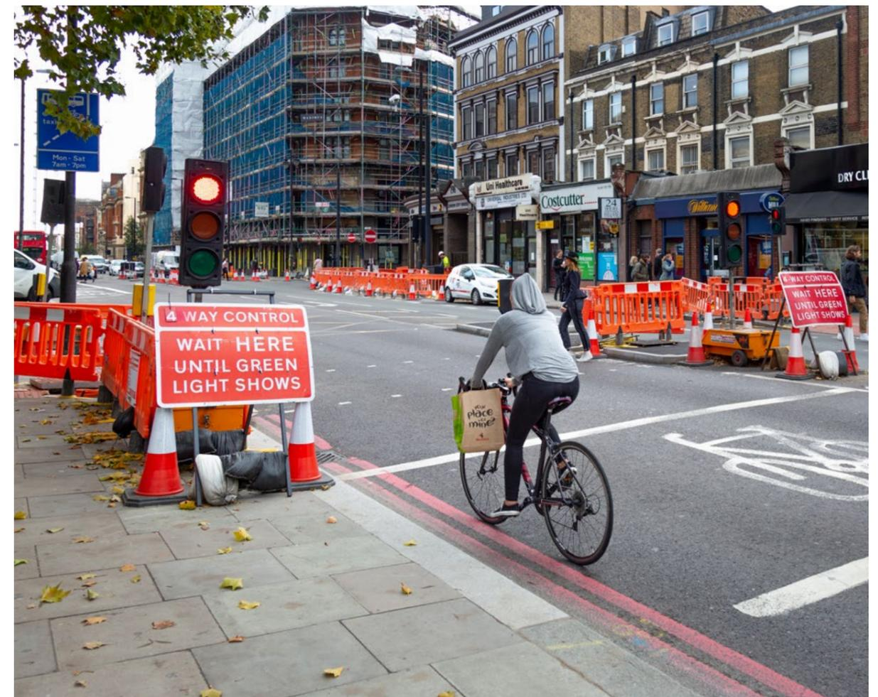
Ensure signal heads and 'Wait here' signs do not prevent cyclists using advanced stop lines
